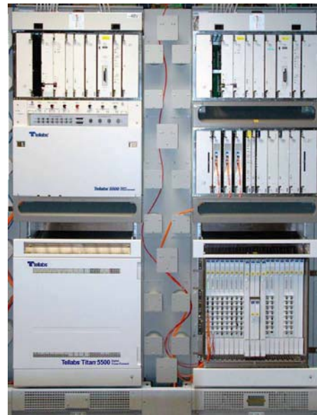
Tellabs Titan 5500 Digital Cross-Connect System Consolidated Core Switch (CCS) Rack
